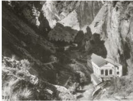
Hydroelectric plant Gampel 1898
